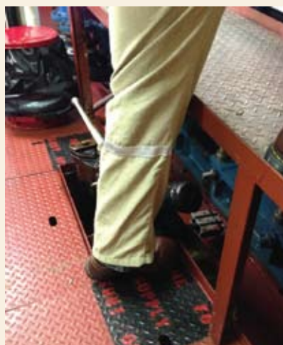
Another view of unstable and inadequate footing that resulted in the accident
